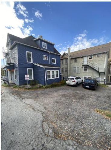
Image 6: Back portion of site
